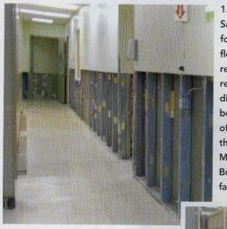
1. Damage from Sandy's three-foot-high floodwaters required the removal and disposal of the bottom half of the drywall throughout Mini-Circuits' Brooklyn, NY facility.
